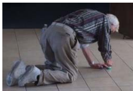
Chuk cleaning grout in the breezeway.
