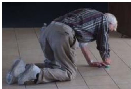
Chuk cleaning grout in the breezeway.
