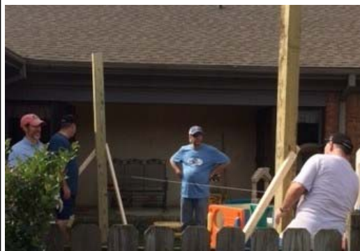
Jeff, Mike, Doug, and Bill installing posts for the swing set in the nursery playground.
