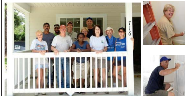
Painted walls and installed soffit while working with Habitat for Humanity.
